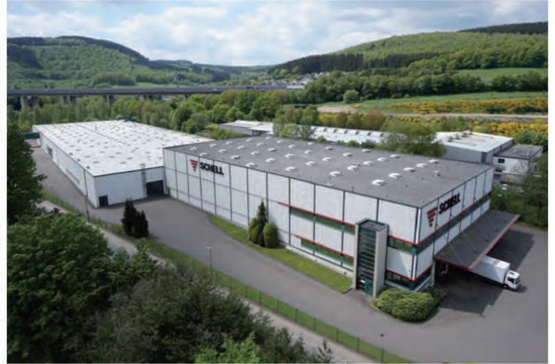
Plant 2 Production with logistics centre
